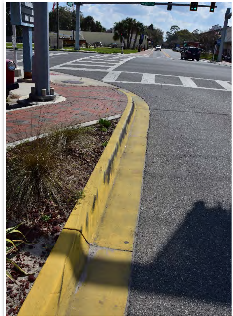
Northeast corner of US 19 at Citrus Avenue looking south showing tire scuff marks over 20 feet away from the intersection.
