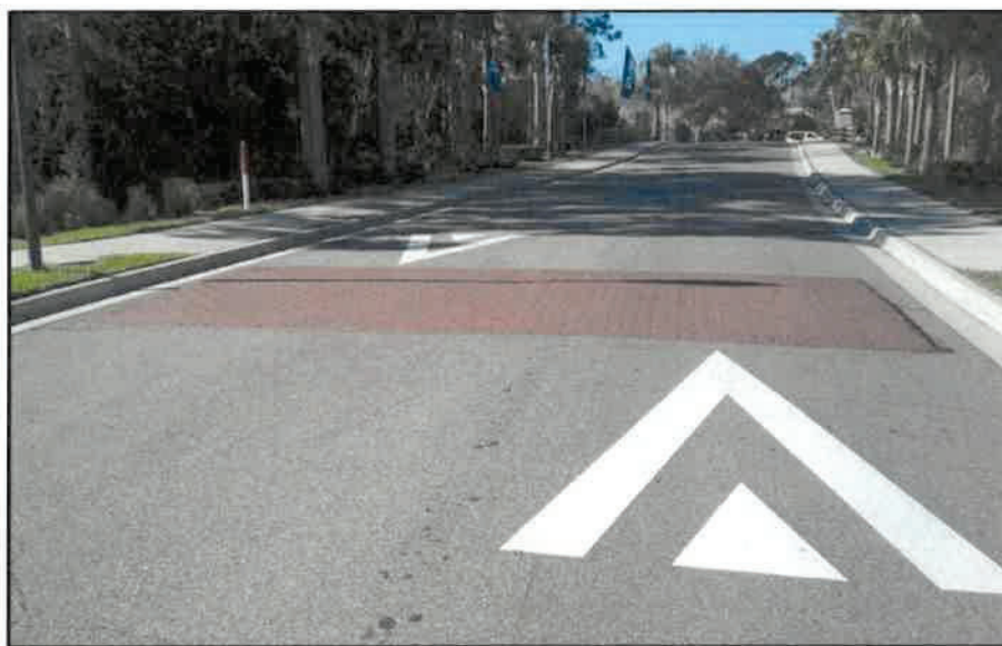
Inside Loop Road, Orange County, Florida
