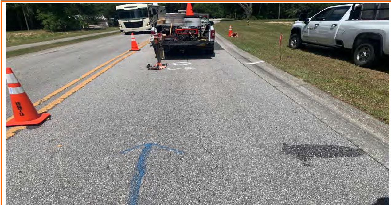
Core Location C-2 with water line markings
