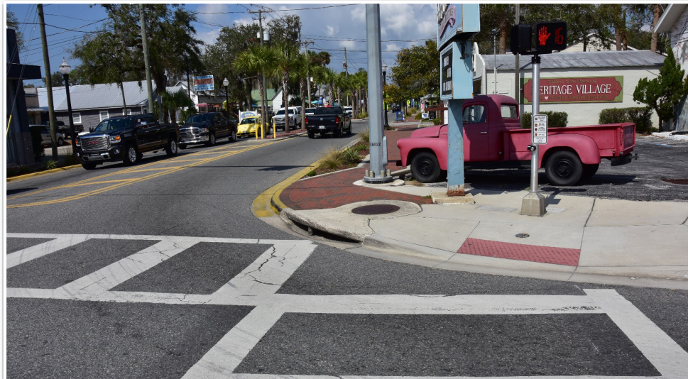
Northeast corner of US 19 at Citrus Avenue looking north showing tire scuff marks on the curbline and drainage inlet.
