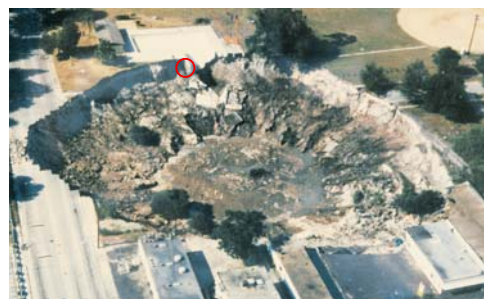
Left: This huge sinkhole opened up in Winter Park, Florida in May, 1981. Notice the four lane road for scale. The red circle in the upper left marks two people. Photo—Florida Geologic Survey
